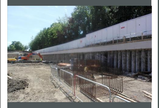
The contract, led by Henry Construction, was to form a levelling coat of Shotcrete over the contiguous piles of a basement in this new development.
